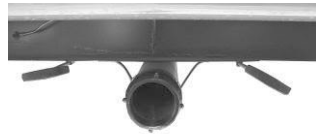
Black/Grey tank drain & valves
