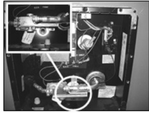
Water heater drain plug
